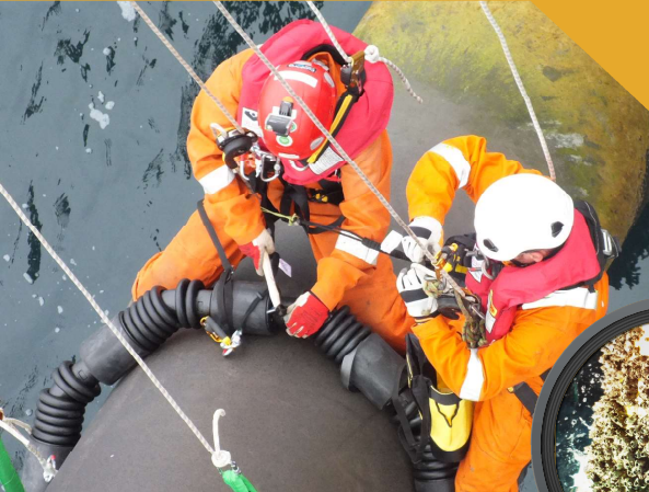
MGP- i installation in the North Sea
