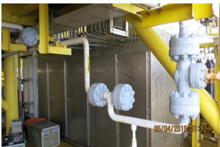
Dong Do Platform: Gas Line after coating
