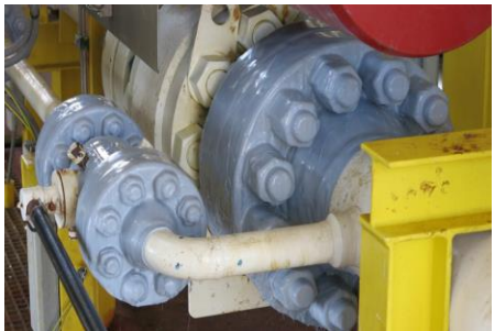
Thang Long Platform: Pig Launcher after cleaning and coating
