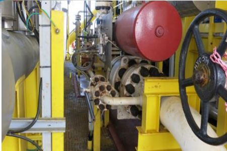
Thang Long Platform: Pig Launcher before cleaning
