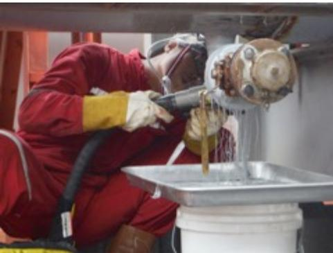
Oxifree coating in progress on a selected flange on the FPSO deck
