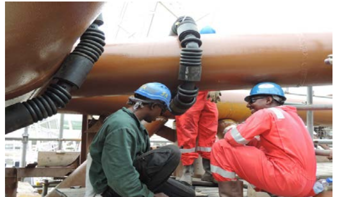
The tagged MGP products were then, installed onto the assigned jacket members.
