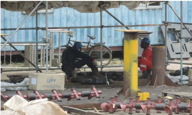
Prior to installation, the MGP products assembled and tagged with the assigned jacket members at the yard.
