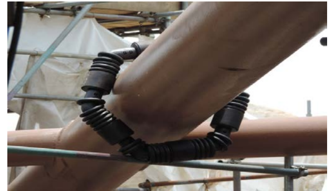
The latest MGP-AI product is specifically designed with more rubber discs on the rigid connectors, to withstand impact from harsh weather condition and its surroundings at the splash zone area.
