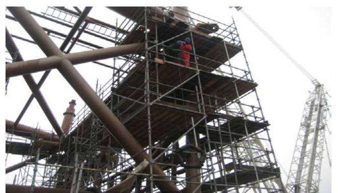
Despite the obstructions on the jacket structure, using rope, the MGP products were lifted up and installed at the designated members.
