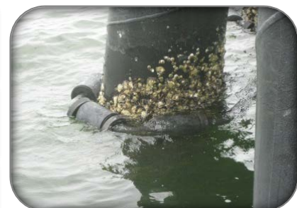
MGP-W SC working on an existing steel pile jetty
