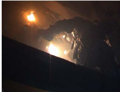
6. Underwater dry welding inside habitat
