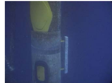
8. Jacket leg after repair
