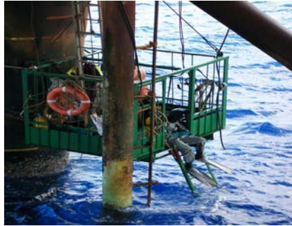
2. Preparation & Deployment of divers
