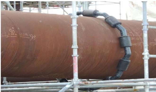
The MGP-SC product is designed with rubber disc that moves along the rigid connectors, to self-clean and prevent marine colonisation on itself, prolonging its service life span.
