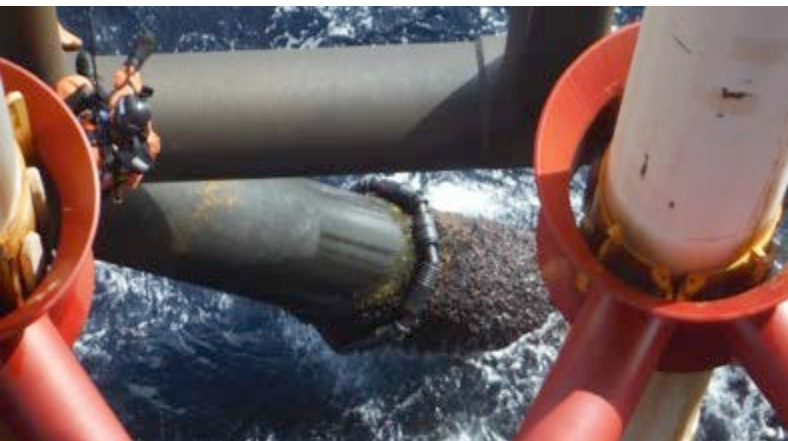
VDM 1-5 - During Installation
