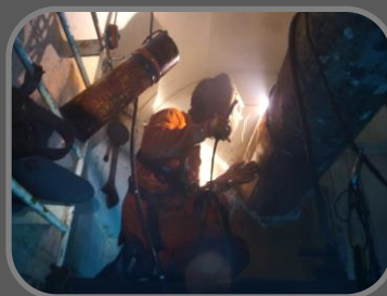
REPAIR IN PROGRESS Trained and certified welder diver performing Underwater Dry Welding
