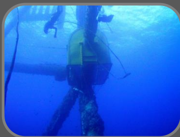
CUSTOM-BUILT HABITAT Custom fit habitat for underwater welding repairs
