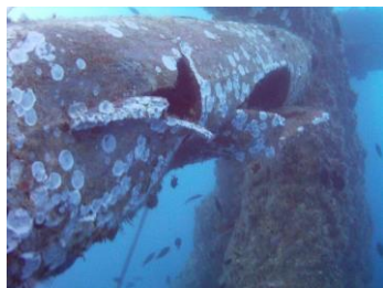
1. Defect on structural member
