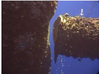
1. Damage at main leg
