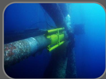
REPAIRED AND REINFORCED Underwater Dry Welding completed and coated
