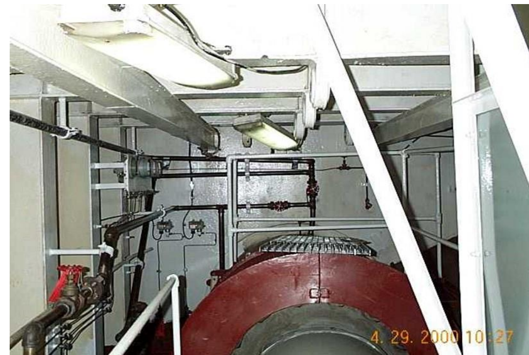
The finished Port Shaft Alley bilge area
