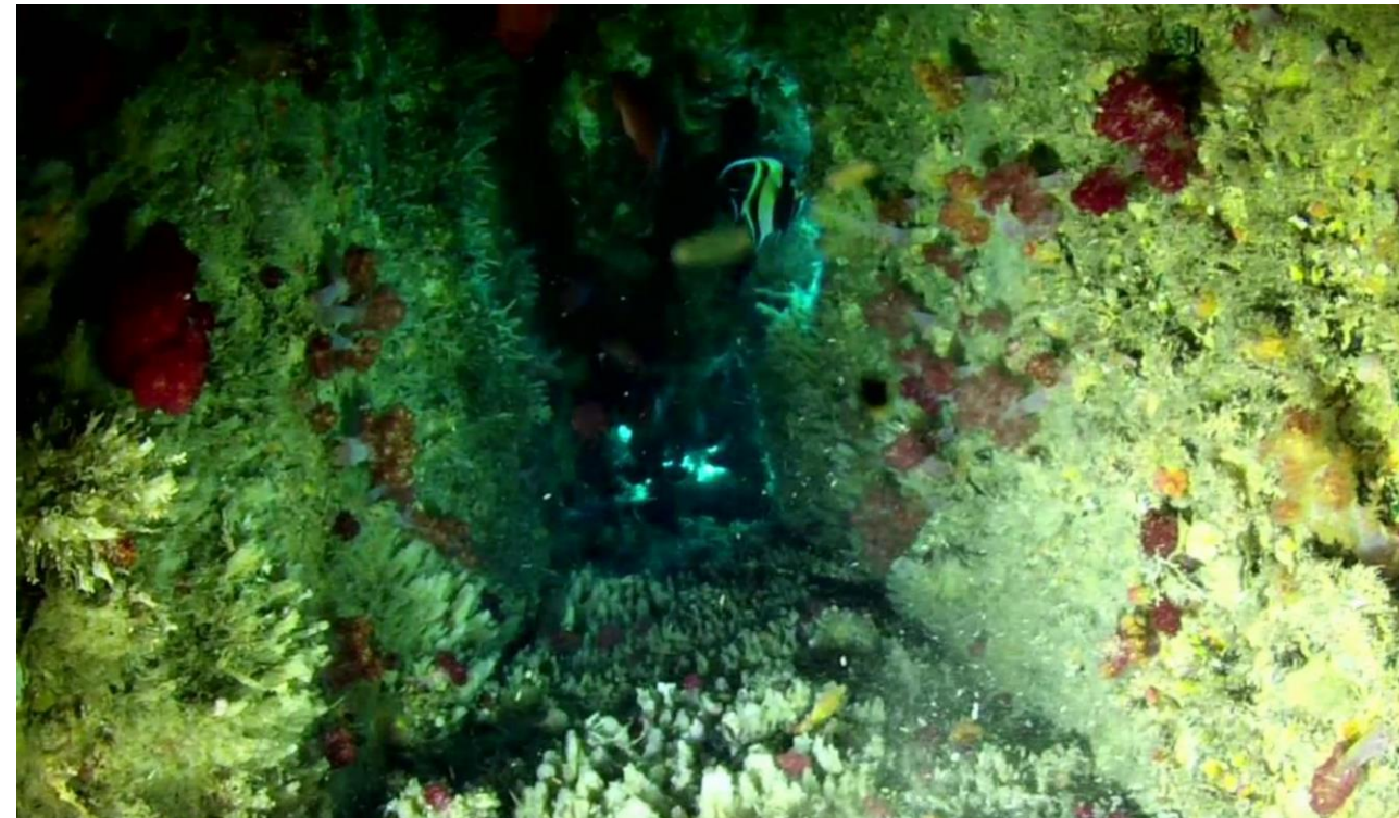
Fairlead internal BEFORE Caviblaster cleaning
