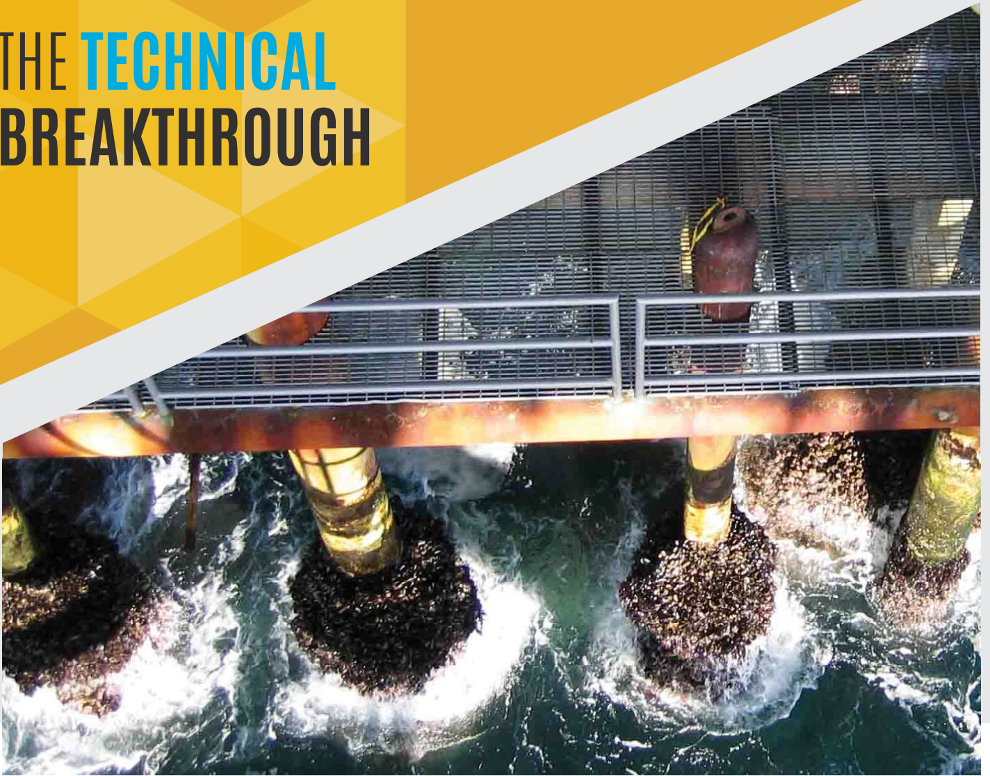
Prolific marine growth on offshore structure
